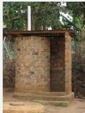
Fossa Alterna spiral toilet in Muteesa P/S
